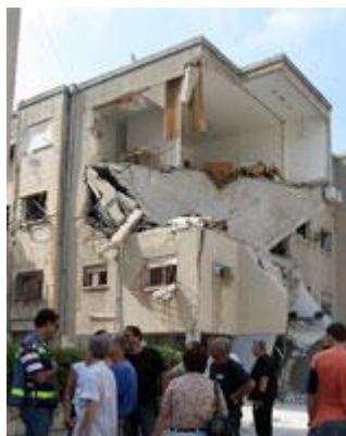
Israelis stand outside a destroyed building in Bat Galim neighborhood of Haifa, Tuesday, July 18. Hezbollah has continued to fire rockets at northern Israel.
